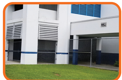
New 6 foot chain link fence at Miramar High School.
